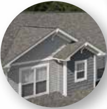
Roofing and Ventilation
